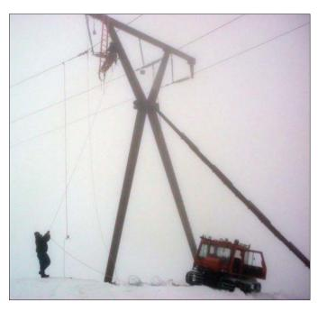
often causes them to fall into our lines. That same heavy snow and ice can build up on our lines and structures causing them to fail as well. Deep snow buries equipment making it difficult to find, let alone access. Strong winds may blow trees into our lines or severely reduce visibility.
