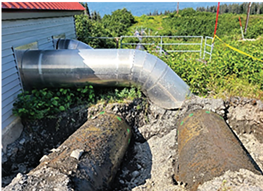
Left, Solomon Gulch penstock excavated for thickness measurement
