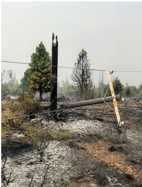
A 2018 wildfire destroyed the electric distribution system serving Eagle Lake in Northern California, leaving about 1,000 people without power. PHOTO COURTESY OF LASSEN MUNICIPAL UTILITY DISTRICT
