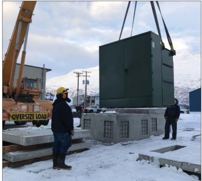
Left, crews replacing conductor to a newly set pole on Kobuk Drive Above, crews installing a new transformer at Silver Bay Seafoods
