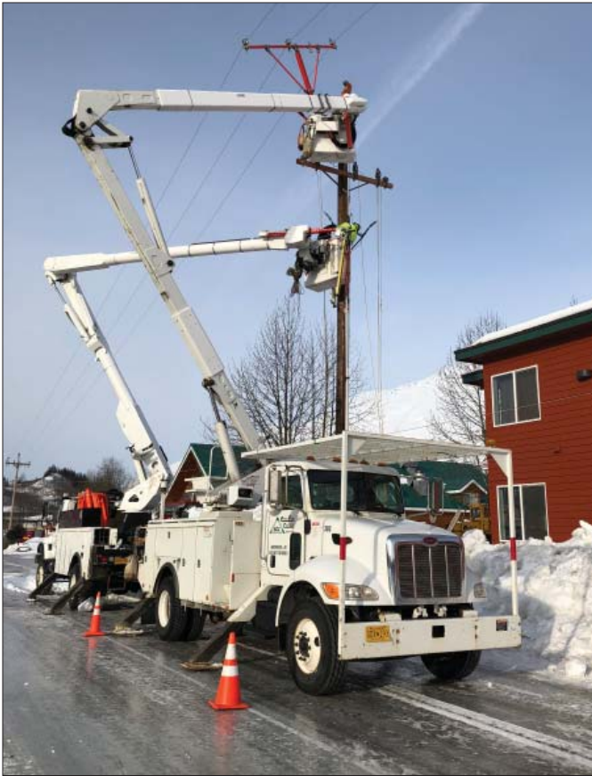
Left, crews replacing conductor to a newly set pole on Kobuk Drive Above, crews installing a new transformer at Silver Bay Seafoods
