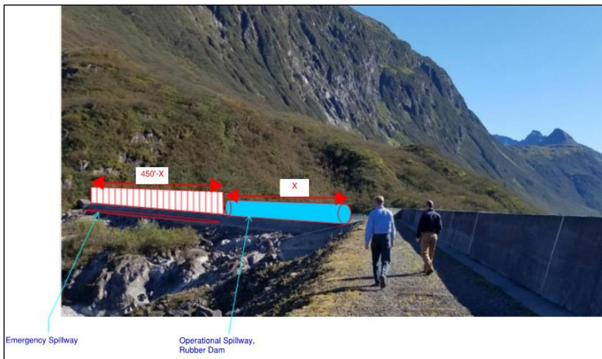
**Figure 4-8. Conceptual sketch of a compound spillway**
