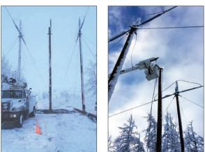
extreme icing conditions east of Thompson Pass resulted in physical damage to three transmission line structures. Above are pictures showing the repair of one structure where the center pole broke due to extreme ice loading. Despite the frost and ice difficulties, we were comforted this winter with few avalanche risks in Thompson Pass after the 2014/2015 relocation of the line from an avalanche prone area to safer ground.
