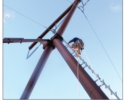
Glennallen Lineman, Ryan Cook, climbs a T-Line structure in Thompson Pass to make repairs
