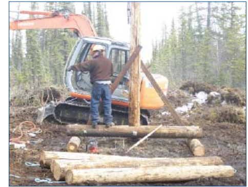
Example of a Bog Shoe structure
