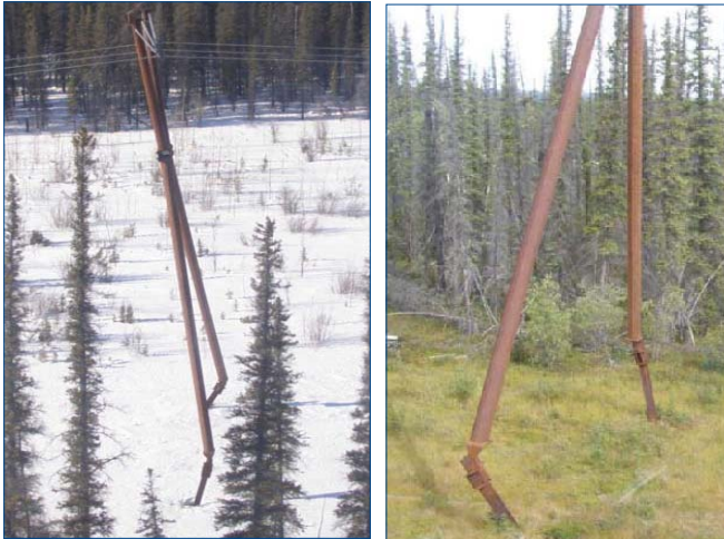
Jacked Transmission Structures
