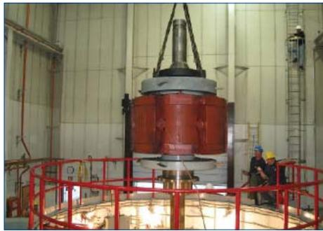
**Rotor clear of stator**
