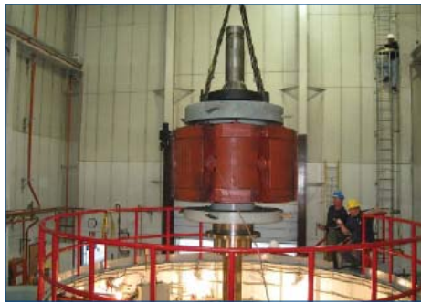
Rotor clear of stator
