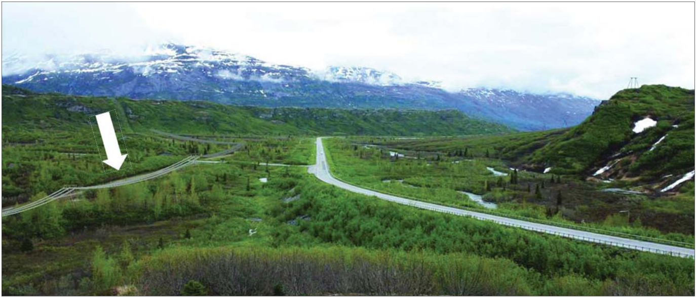
Left, routing map of the Thompson Pass area. This clearly demonstrates that the CVEA transmission line and towers are currently in the avalanche trouble zone. Above, a rendering of the Thompson Pass area showing option 2A; the proposed route west of the Richardson Highway. Courtesy Dryden & LaRue, Inc.
