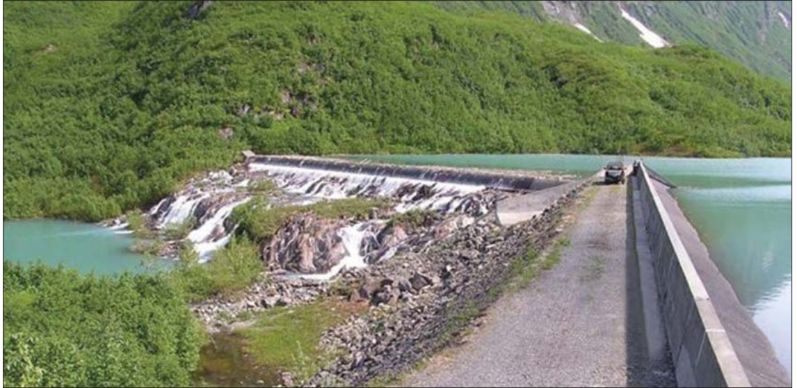
Solomon Lake Dike and Spillway; illustrates a full lake with water overtopping the spillway.
