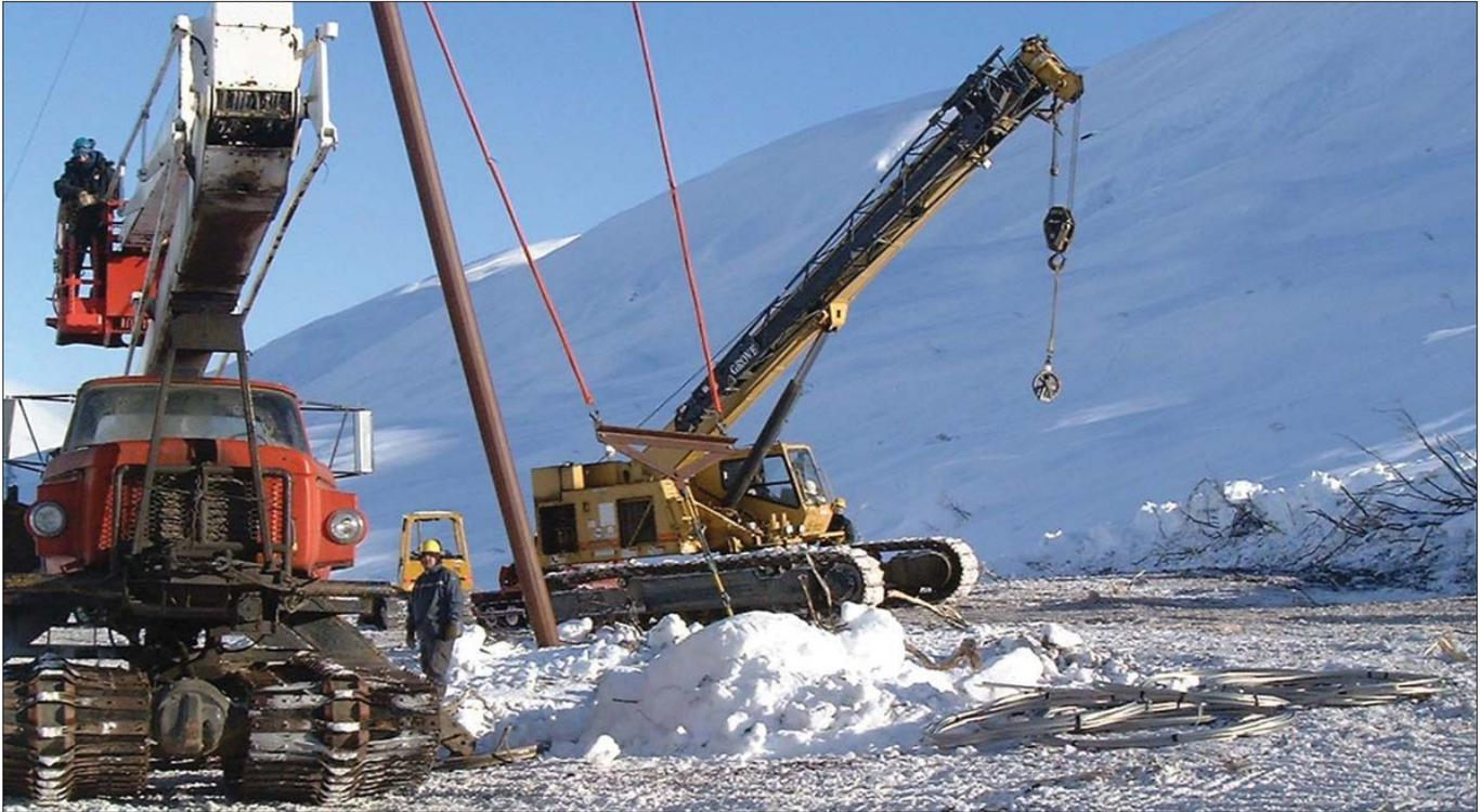
**Above:** City Electric work crews on site on Thompson Pass in 2003, as they worked to replace Structure 46-2 which had been taken out by an avalanche. **Below:** Looking Southbound down the T-Line at Structures 46-3, 46-2, and 46-1.
