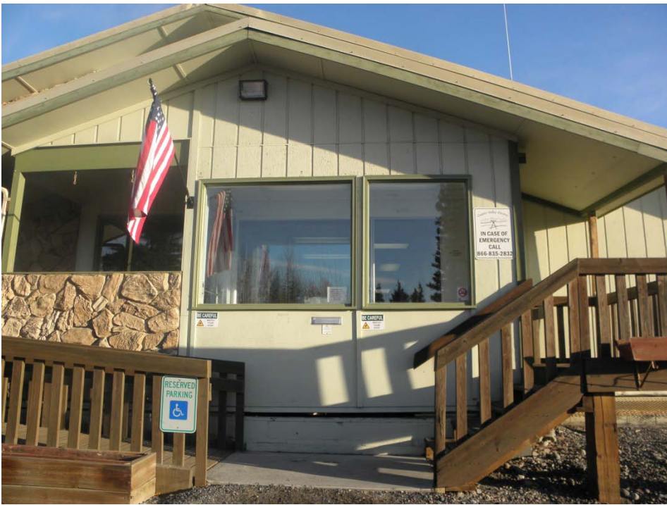
Front View of Entry Porch
