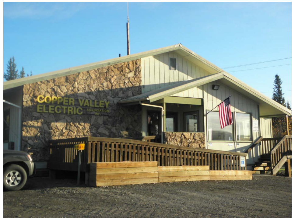
Full View of Front of Building
