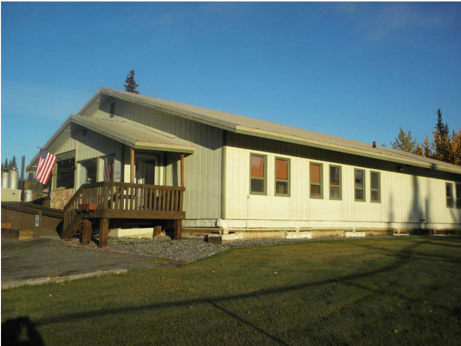
Side View of Building
