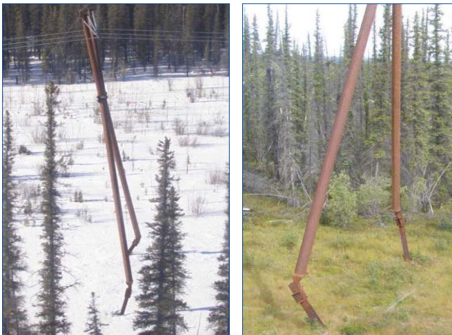
Jacked Transmission Structures
