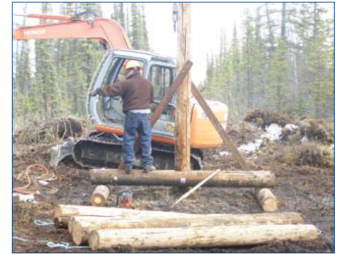
Example of a Bog Shoe structure
