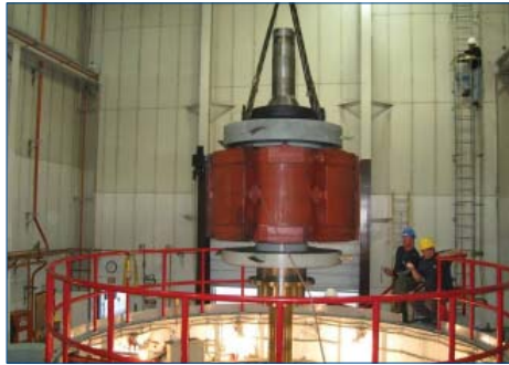
Rotor clear of stator
