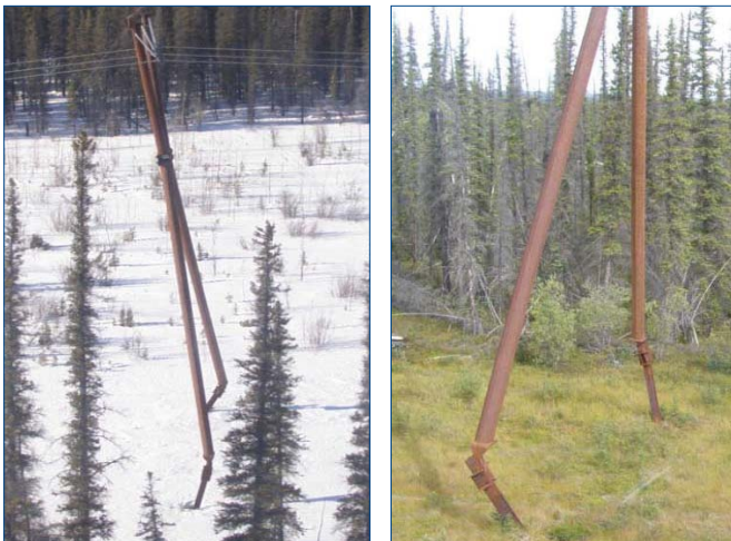
Jacked Transmission Structures
