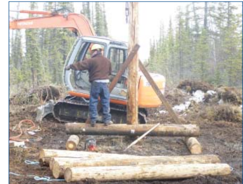
Example of a Bog Shoe structure
