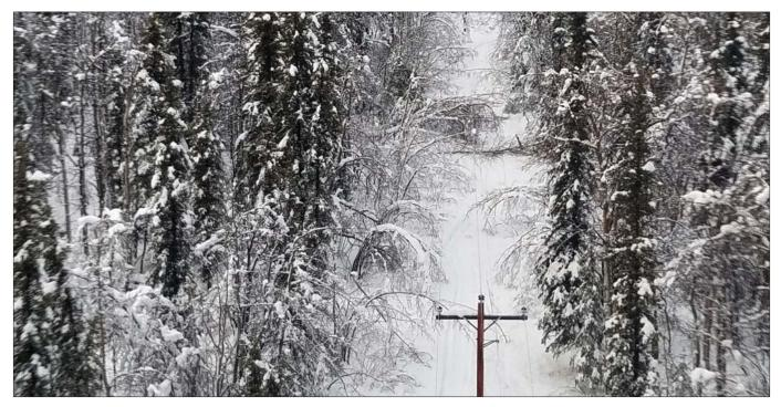
Above, heavy, wet snow forced many trees from outside CVEA's right of way into this small section of power lines
