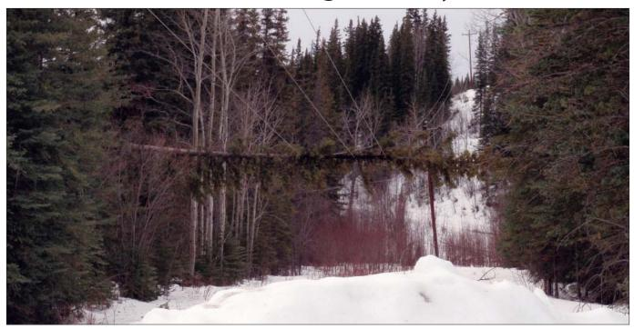
Above, a tall tree from far outside CVEA's right of way in the Copper Basin fell into the power line
