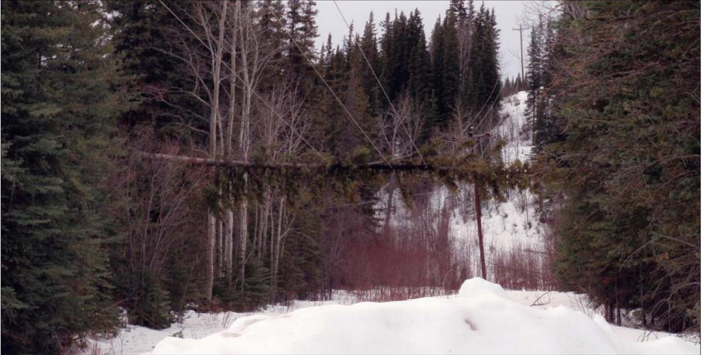
**Above, a tall tree from far outside CVEA's right of way in the Copper Basin fell into the power line**
