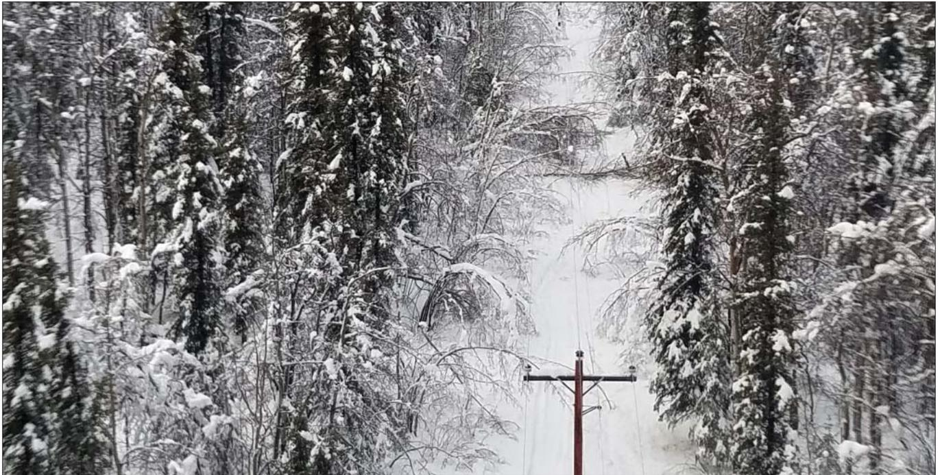
**Above, heavy, wet snow forced many trees from outside CVEA's right of way into this small section of power lines**
