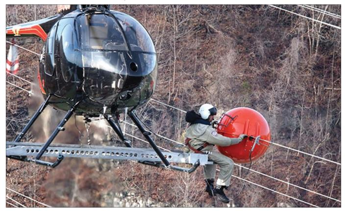
Above, a specially trained lineman performing marker ball replacement on a power line from a platform attached to a helicopter
