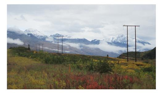
thanks to completion of the effort to re-route nearly four miles of the line in Thompson Pass out of a high risk avalanche zone. Since being built in the early 1980s, avalanches destroyed portions of the line five times with a total cost to repair of over \$2.675 million.
