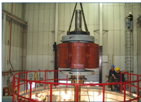
Rotor clear of stator
