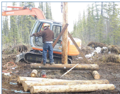
Example of a Bog Shoe structure
