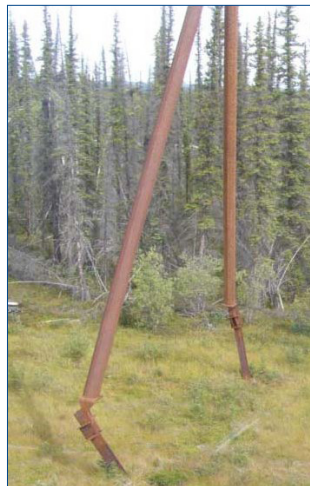
Jacked Transmission Structures
