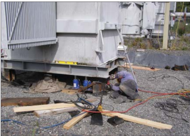
Top Left: Using heavy duty jacks to jack up the reactor. Above: Dan Dempsey, Chief Plant Operator for the diesel plants, working on the underside of the reactor. Top Right: Completed Reactor Repair Project. Bottom Right: Plant Operator, Mike Rego, welding one of the components of the structure. Photos by Jimmy McDougald
