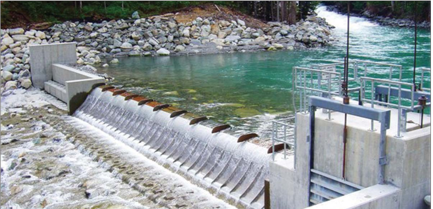
Above, an example of a Run-of-River hydroelectric project, similar to what is proposed for Allison Creek
