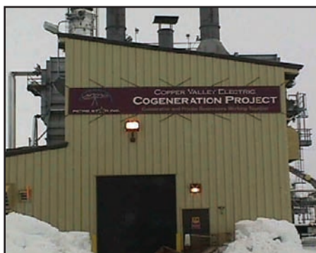
Copper Valley Electric Association Cogeneration Plant, supplying roughly 25% of CVEA's annual generation
