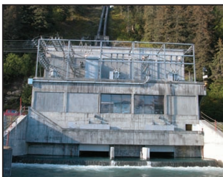
Solomon Gulch Hydroelectric Plant, supplying 60% of CVEA's annual generation
