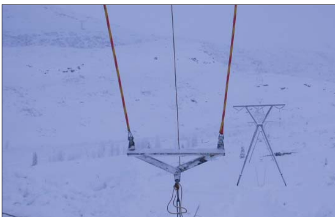
Putting the guy yoke back in place
