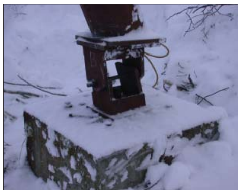
Replacing upper/lower flange assembly and shear pin on the footer
