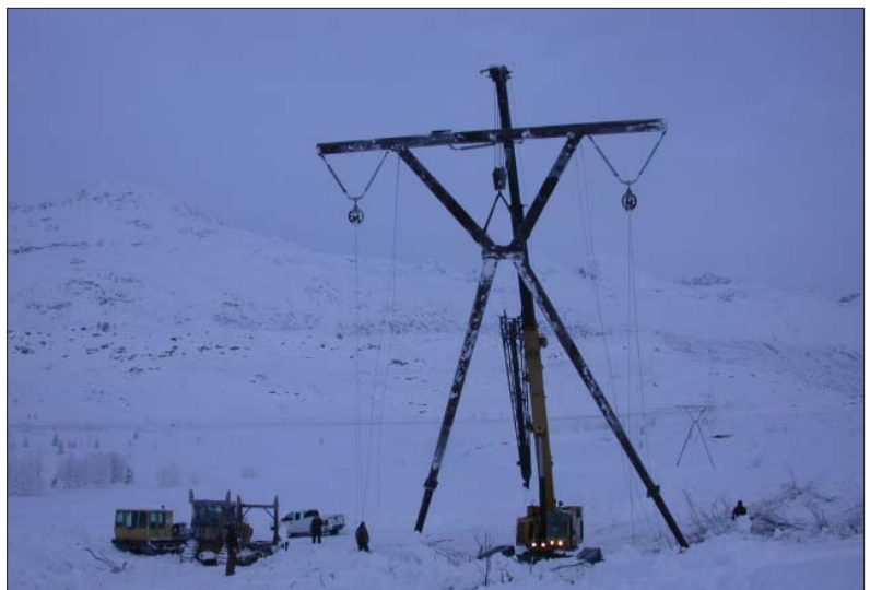
Tower 46-3 successfully back in the air
