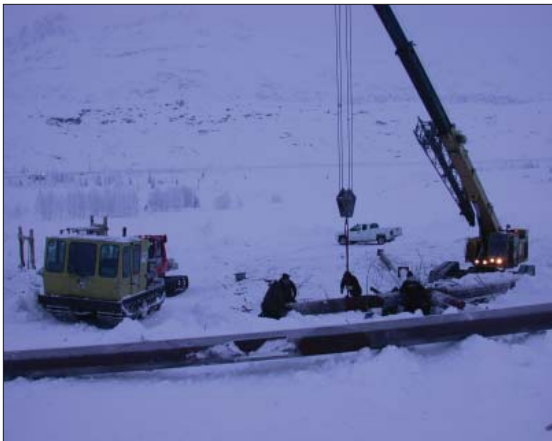
Connecting the tower to the crane
