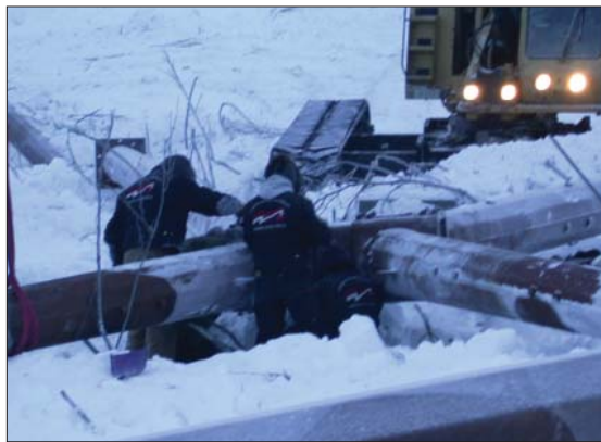
Crew making final adjustments
