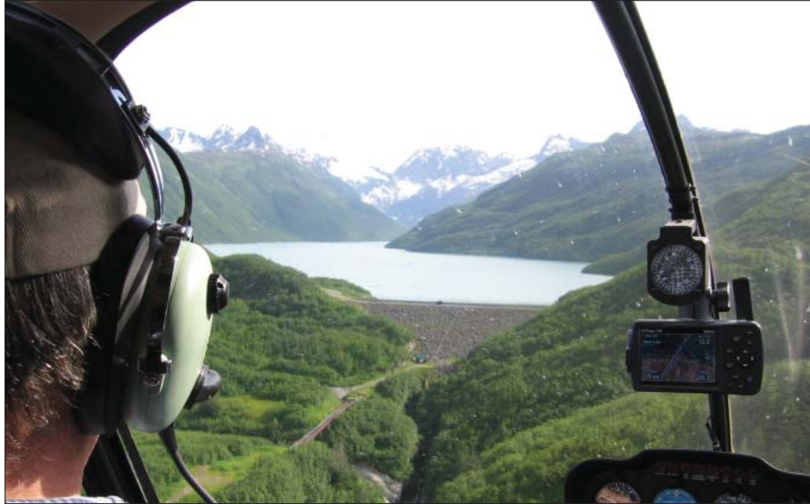
Aerial view of the Solomon Lake Dam from a helicopter
