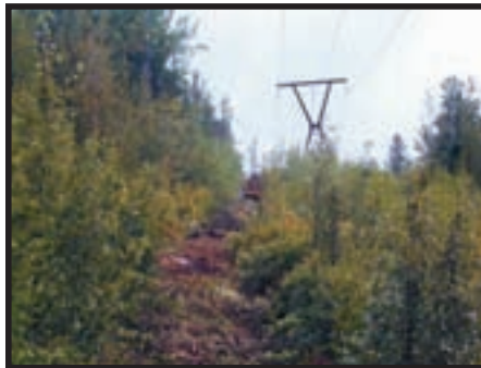
CVEA contractors clear over grown right of way on the transmission line
