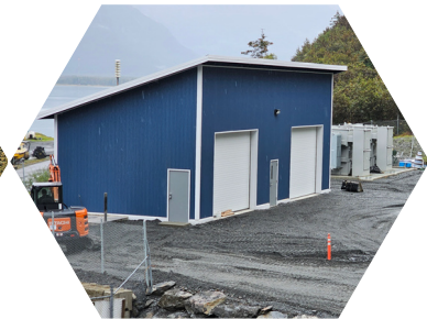
Solomon Gulch Substation
